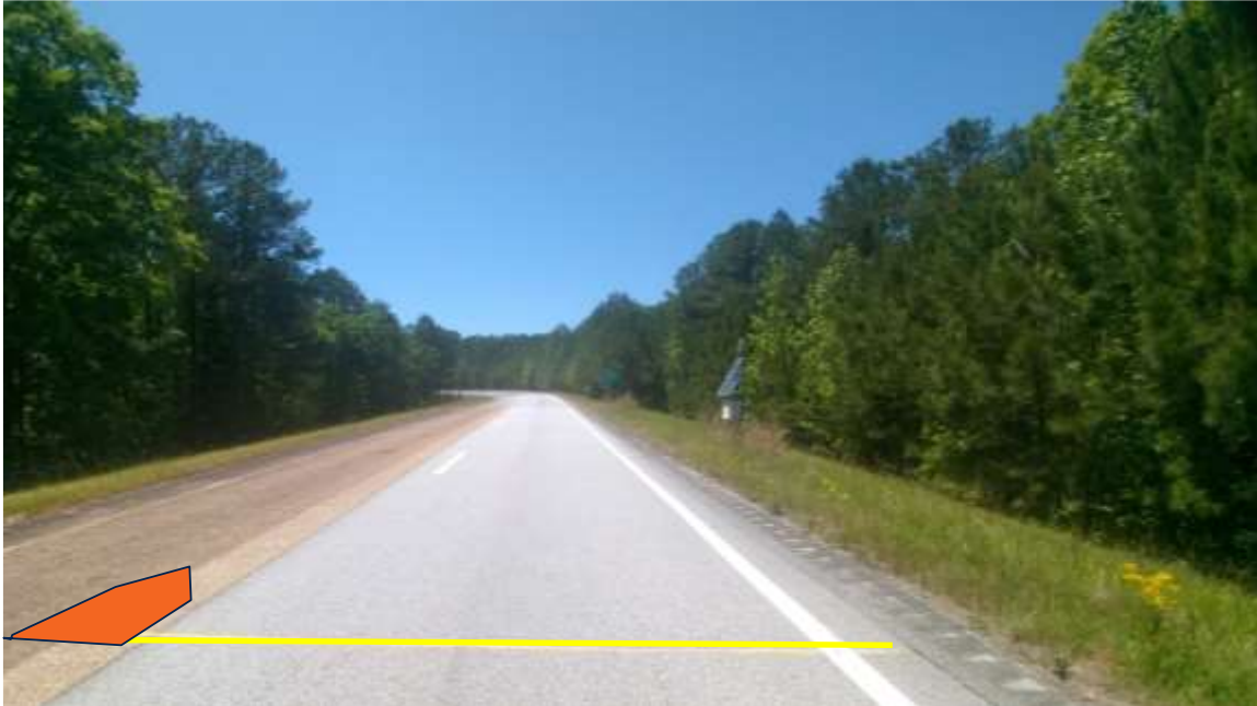
FIGURE 17 Subsection N13-B ARGG, 0.35-inch rutting, 3.1% cracking (April 2024).
