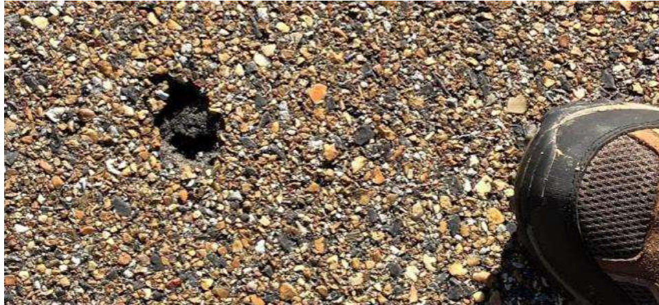
FIGURE 5 Pop-out in Section S2.
