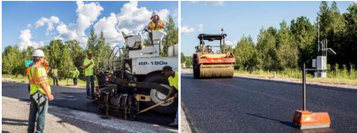
FIGURE 5. Constructing Section S11 with a volumetric mix.
