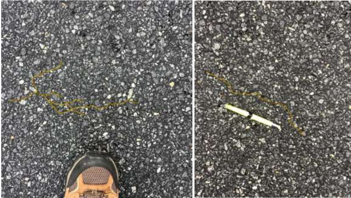
FIGURE 2 Sample cracking in N4 on 1/25/2021 (29.6 million ESALs).
