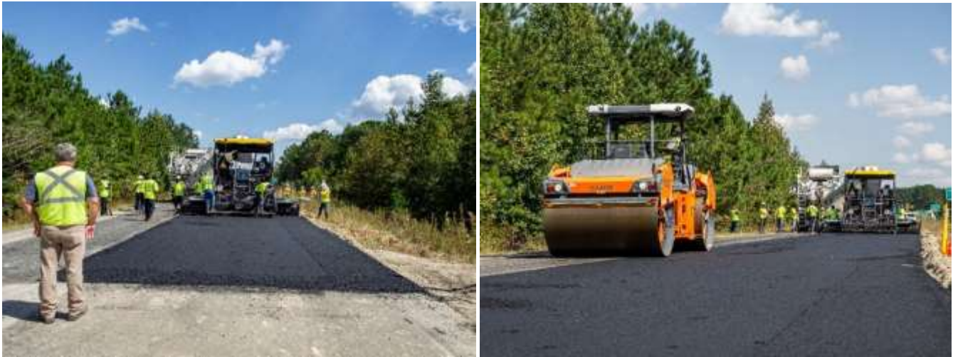
Figure 5. S8 Mix Placement and Compaction
