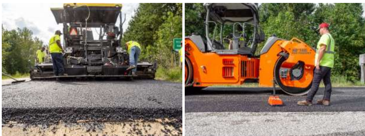
FIGURE 6. Constructing Section N6 with a BMD mix.
