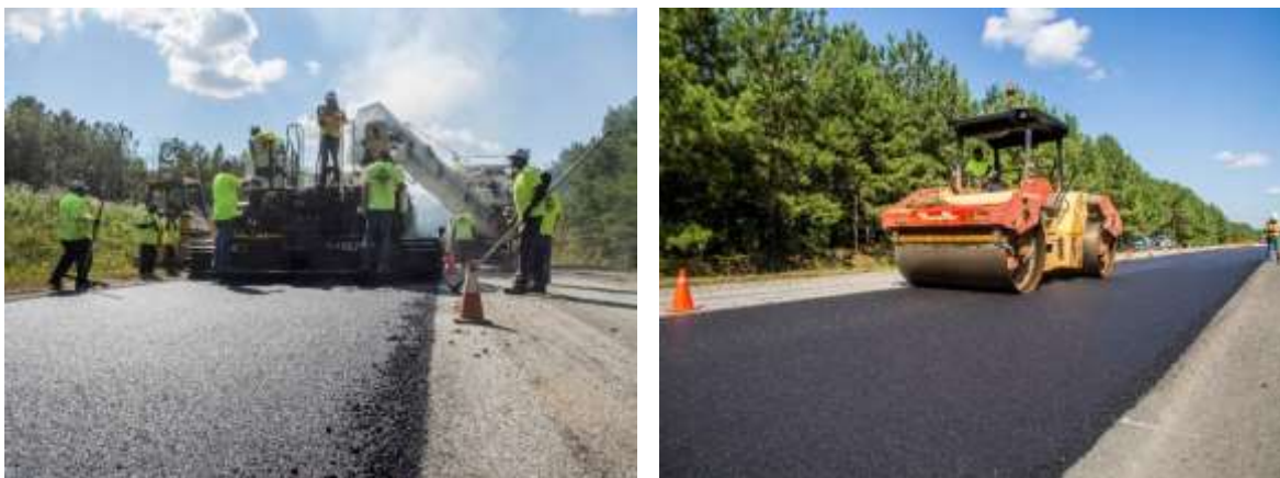
FIGURE 4 Laydown and compaction of S1 surface mix.
