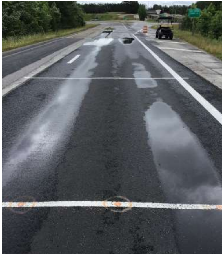
FIGURE 6 Rutting in Section S12 (April 2022).
