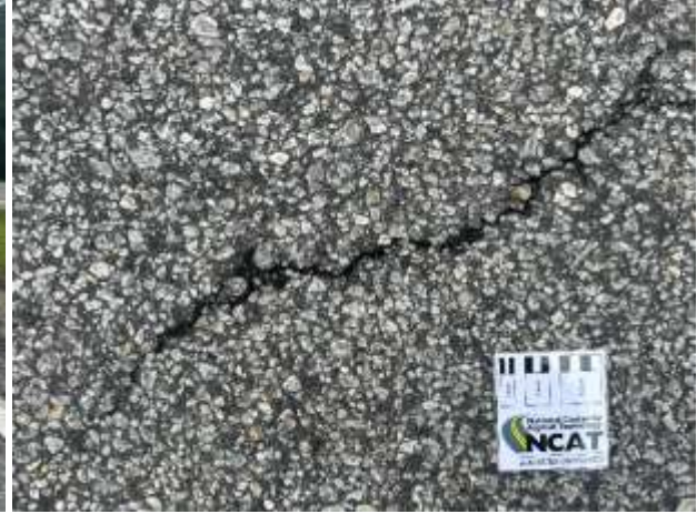
E5A (93.6% of G_{mm} ) representative cracking
